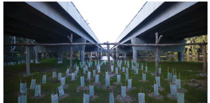
Bonville Upgrade, Pacific Highway - Image Courtesy of Abigroup
